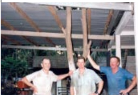
Team Members Underneath The Roof They Built
