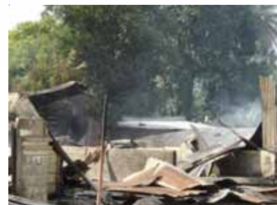
Burnt house in Dili
